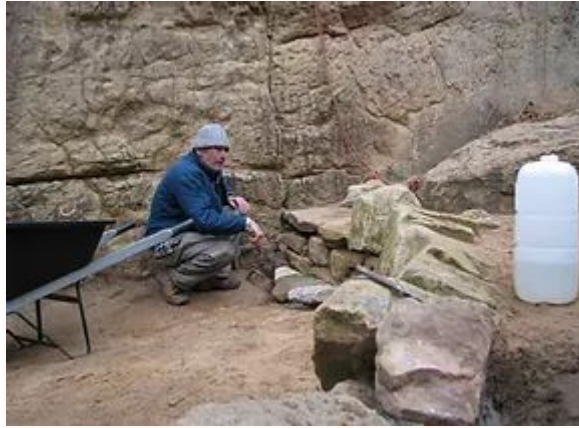
Pic 33. - Stone retaining wall made from local and imported stone to the prevent further erosion at this well known and high traffic area. Work completed by Cliffcare and Parks Victoria and with paid and volunteer efforts. Local climber, steward and volunteer indicating where erosion occurred. Photo Cliffcare Collection.
