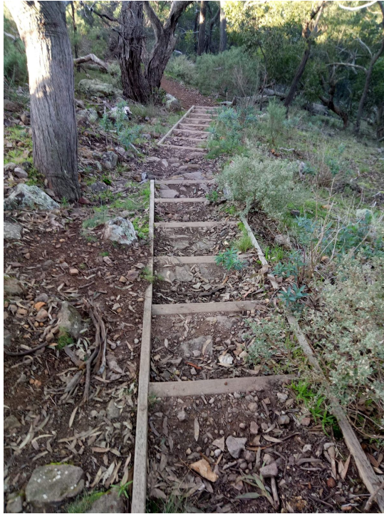
Pic 27. Formalisation and stabilisation of climber access trails at Falcons Lookout performed by Cliffcare volunteers in collaboration with Parks Victoria staff - critical to the prevention of erosion in well known sites and high traffic areas. Photo Aaron Wain.
