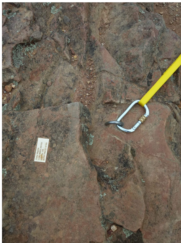
Pics 35 and 36. - Parks Victoria funded fixed safety anchors installed at Staughton Vale, Brisbane Ranges to protect trees, prevent erosion and improve safety at this site. Work completed by Cliffcare and Parks Victoria and with paid and volunteer efforts. Photo Cliffcare Collection.
