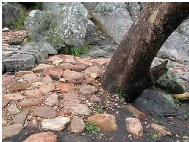
Pic 32. Formalisation and stabilisation of cliff base staging after completion at Bushrangers Bluff formation at Djurite / Mt Arapiles - local and imported stone used to prevent further erosion at this well known and high traffic area. Work completed by Cliffcare and Parks Victoria and with paid and volunteer efforts. Local climber, steward and volunteer indicating where erosion occurred. Photo Cliffcare Collection.
