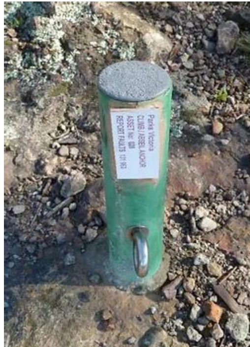
Pic 34. - Parks Victoria funded belay anchors installed at Werribee Gorge to protect trees and improved safety at this well known and high traffic area. Work completed by Cliffcare and Parks Victoria and with paid and volunteer efforts. Photo Cliffcare Collection.
