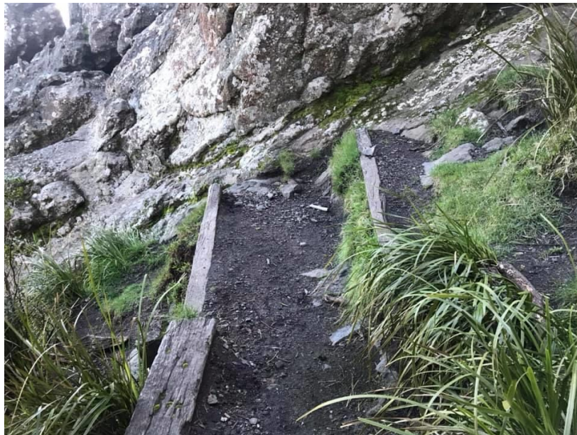
Pic 12. - In 2004 collaboration between VCC, Cliffcare and Parks Victoria saw railway sleepers placed into the soil of the Omega Block gully at Camels Hump, to prevent erosion and improve safety at this site. Work completed by Cliffcare and Parks Victoria and with paid and volunteer efforts. Photo Peter Upton.
