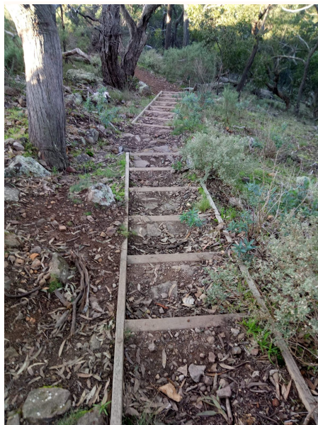
Pic 38. - VCC, Cliffcare and Parks Victoria constructed steps at Falcons Lookout, to prevent erosion and improve safety at this site. Work completed by Cliffcare and Parks Victoria and with paid and volunteer efforts. Photo Aaron Wain.
