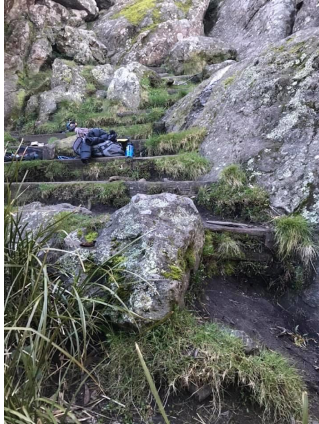
Pic 37. - VCC, Cliffcare and Parks Victoria placed railway sleepers into the soil of the Omega Block gully at Camels Hump, to prevent erosion and improve safety at this site. Work completed by Cliffcare and Parks Victoria and with paid and volunteer efforts. Photo Peter Upton.
