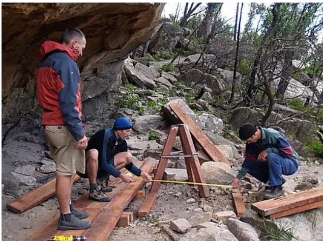
Pic 6 and 7. In 2008 after Aboriginal Surface Scatters were discovered under a climb named “Manic Depressive” at Bundaleer, CliffCare and Parks Victoria’s Cultural Heritage team worked together to create a boardwalk and wooden tripod to protect both this area and the climb above. Photo Credit Cliffcare Collection
