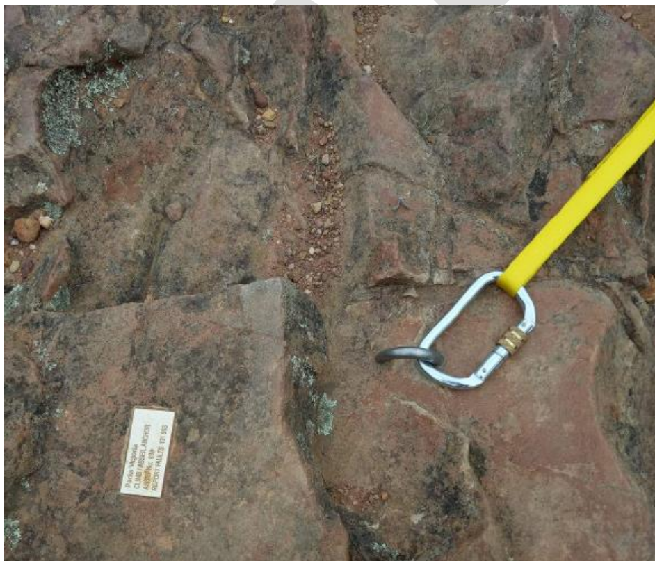
Figure 5 – Parks Victoria funded safety anchor installed at Staughton Vale, Brisbane Ranges to protect trees, prevent erosion and improve safety at this site. Work completed by CliffCare and Parks Victoria. CliffCare collection.
