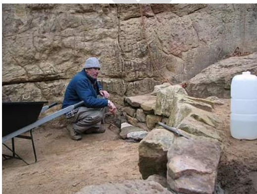
Figure 2: Retaining wall repair at Summerday Valley, 2008
