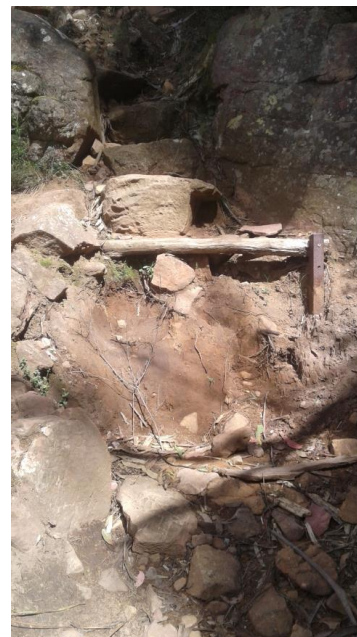
Figure 8: erosion on the approach to the Watchtower (near Halls Gap)
