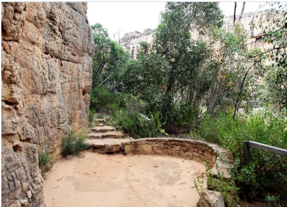
Figure 13 – the base of Back Wall at Summerday Valley. Note the stonework constructed by Parks Victoria and CliffCare at the base of climbs. Note also the wood post and wire fence that separates the public from the regrowth in the valley floor and from the quarry sites across the valley at Wall of Fools.
